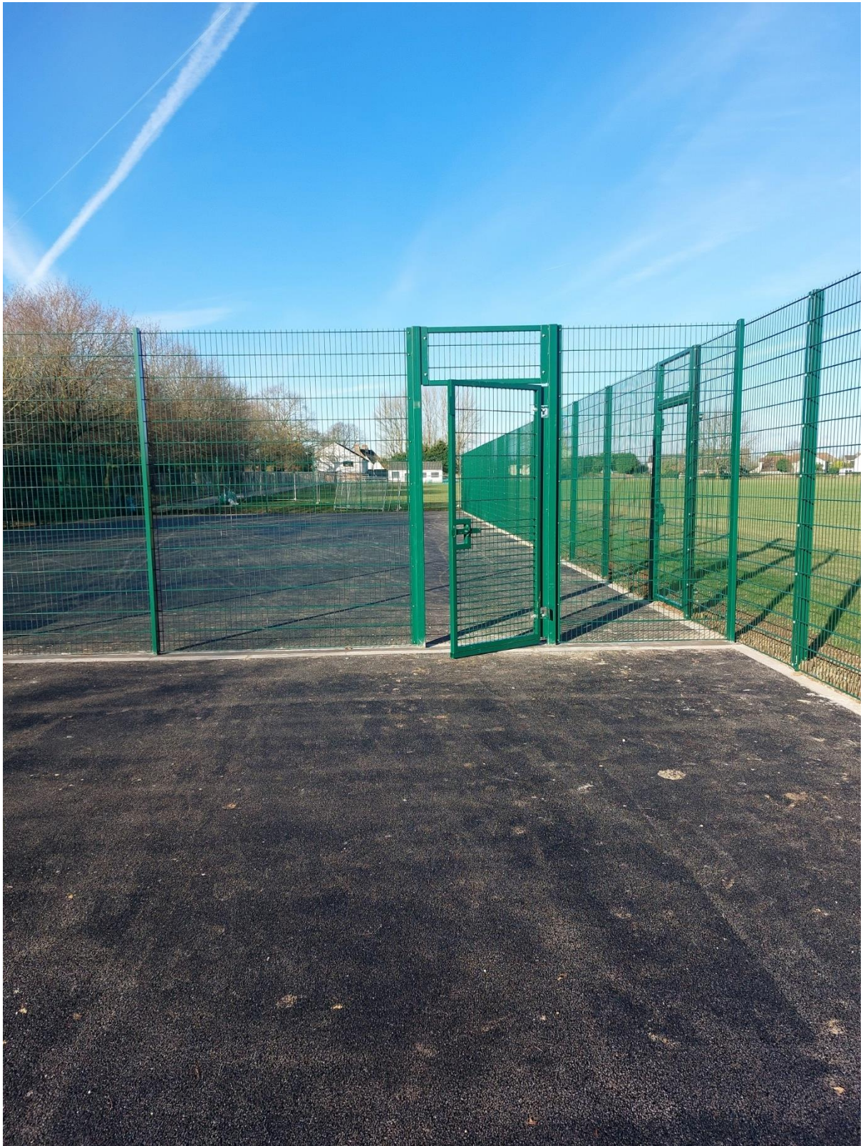
Photo shows the new fencing and gates
